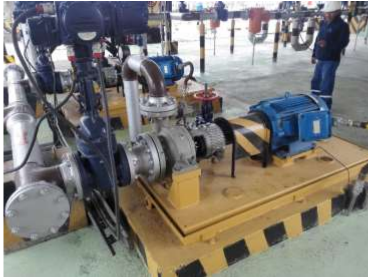
Figura 10: Bombas Booster
