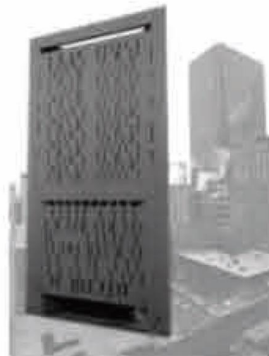
Metropolitan Correctional Center Chicago
