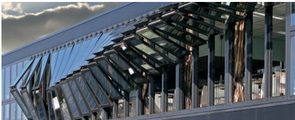
CAFE-RESTAURANT OPEN, AMSTERDAM / by de Architekten Cie
